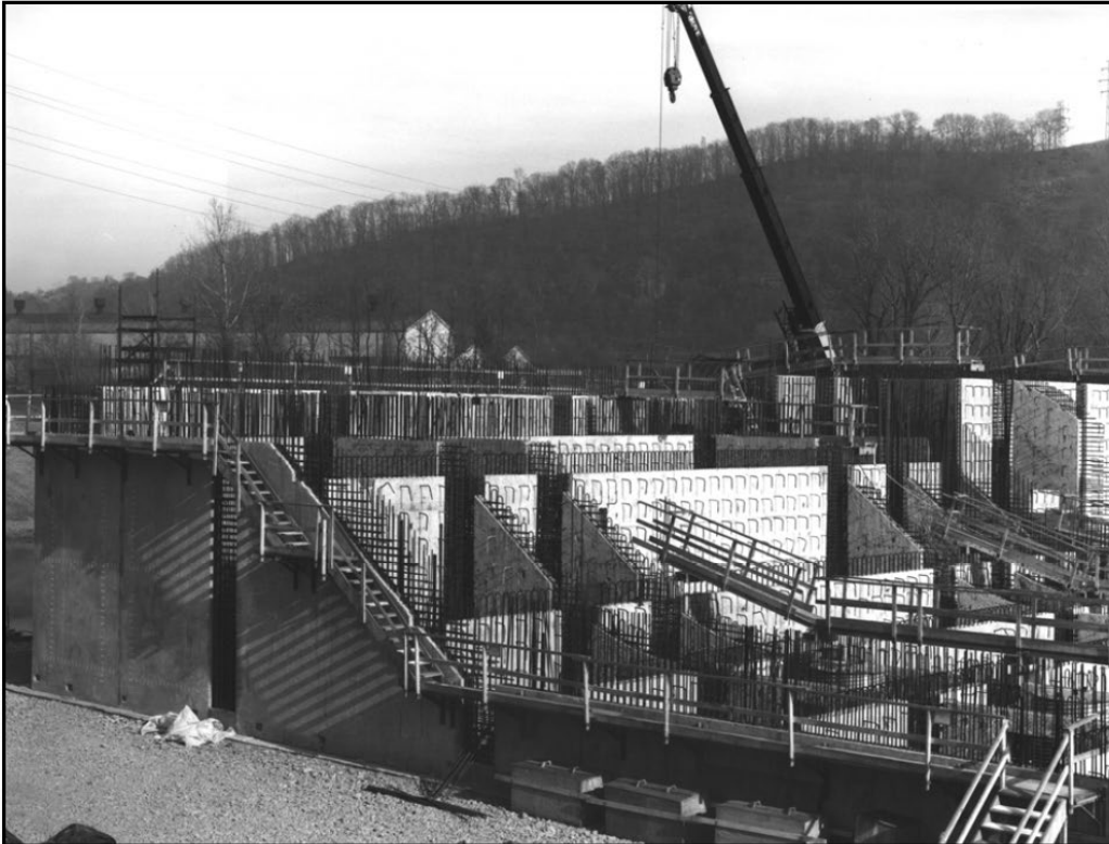
Plate 37. Braddock Dam, Monongahela River. Construction of dam segment in casting basin.
